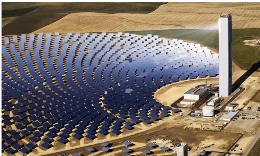
Picture2: A sea of mirrors directs a powerful beam of light toward a solar power tower. (NASA, 2016)
