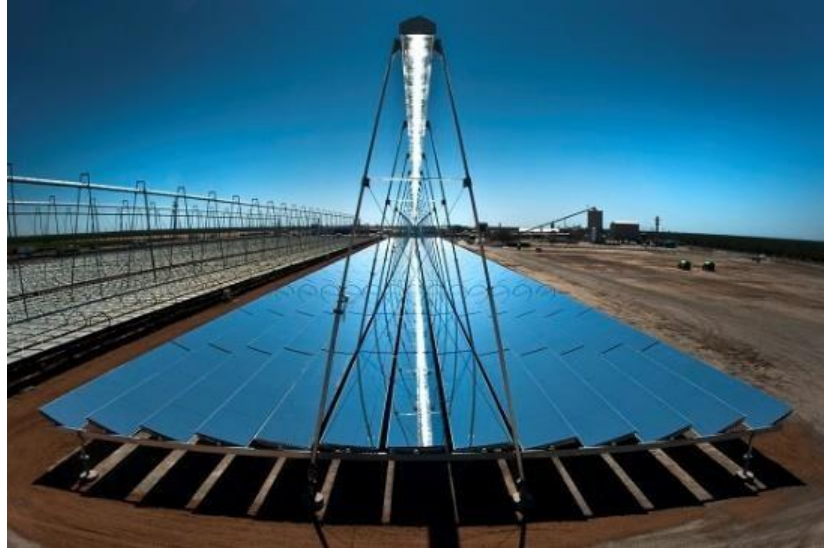
Picture4: A linear Fresnel Reflector (Solar Energy Industries Association, 2014)
