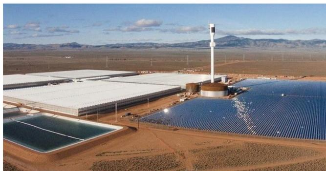
Fig.1. An integrated desalination facility drawing its main electricity from an adjacent concentrating solar power plant (Inhabitat, 2016).
